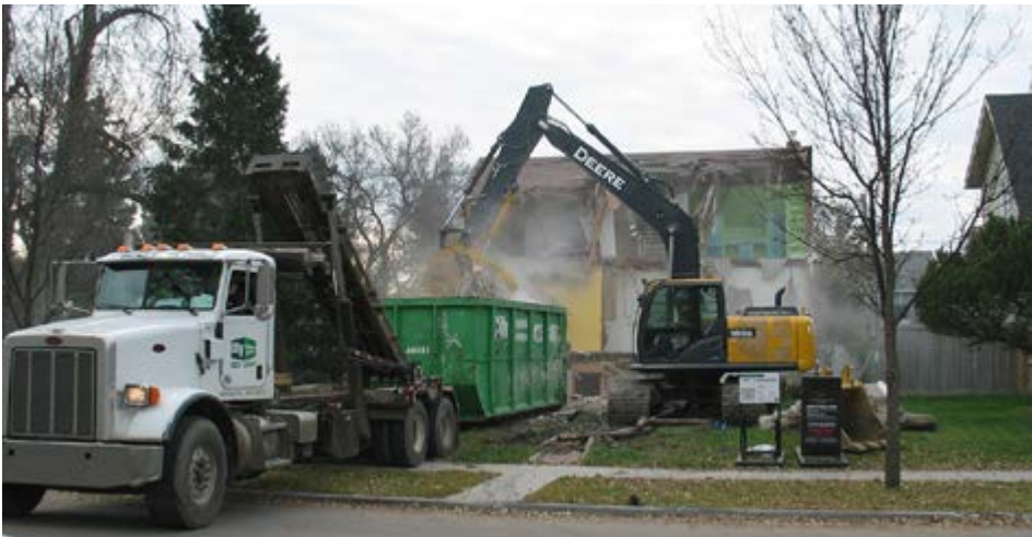
A Parkallen home is demolished ahead of a planned infill construction.
